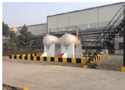
2 x 10m3 - Ammonia Storage & Regassification System - Gold Plus Glass Industry, Roorkee, India
